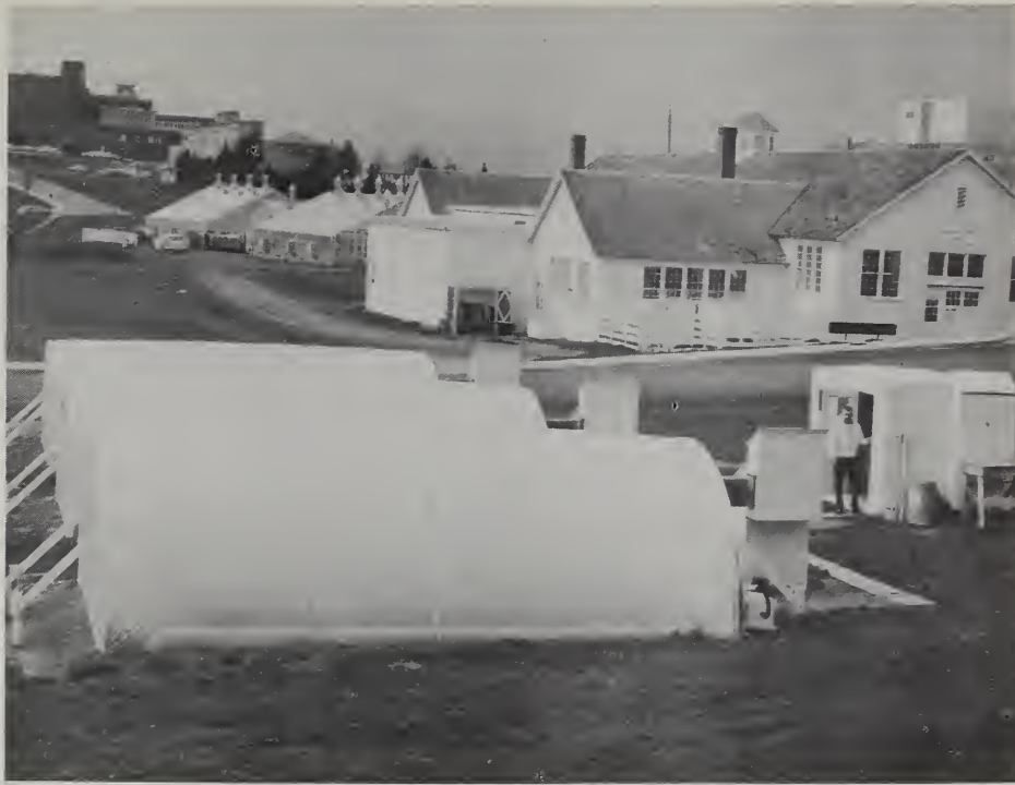
Figure 1.--Air-supported plastic greenhouses in which the carbon dioxide concentration is controlled automatically.
